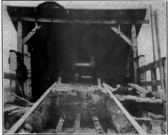
Hoist at Top of Incline
